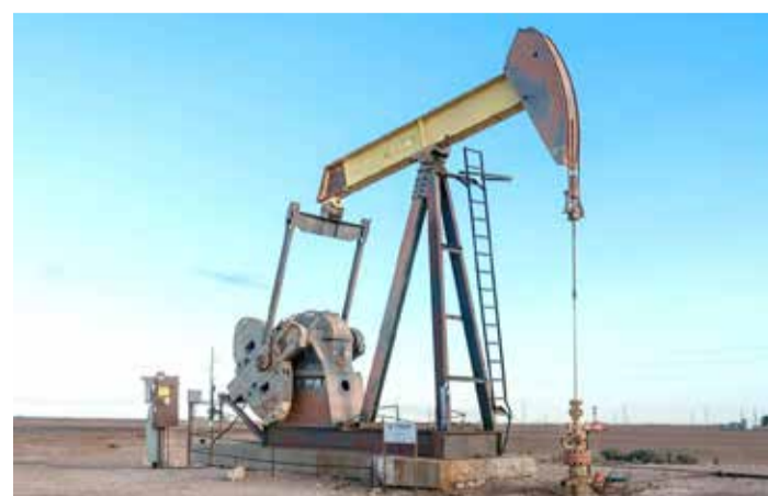
Oil rig and pump of H&P Rig 488 in Stanton, Texas
